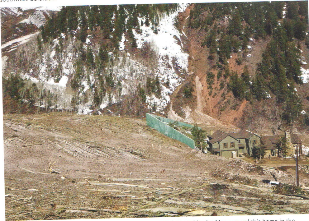
This concrete splitting wedge avalanche diversion structure designed by Art Mears saved this home in the Conundrum Creek valley south of Aspen.
